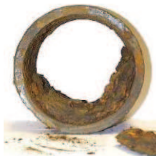
Scaling and Corrosion
